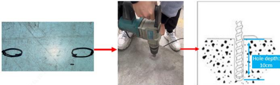
Figure 5-3 Drill Holes
